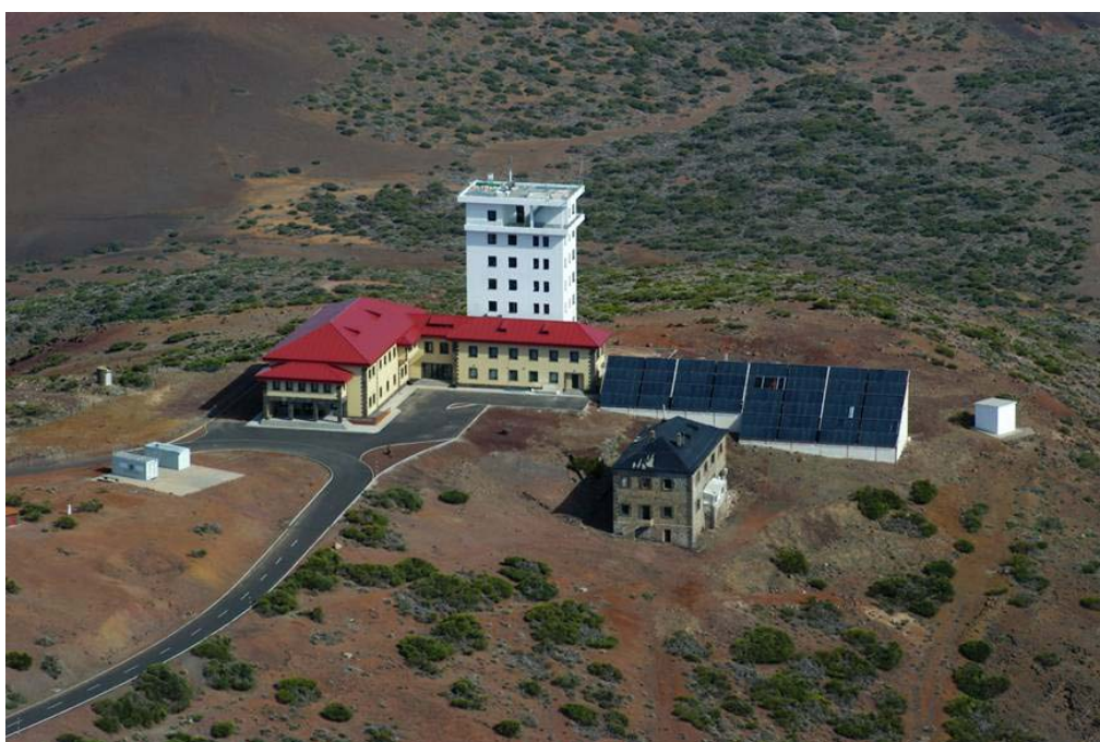
Fig. 3 : Overview on the Izaña observatory buildings. The GAW-related laboratories are located in the upper floors of the tall building. Installations for air intake and meteorological measurements are located on the roof.
